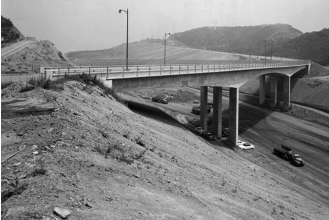
The Mulholland Bridge, completed in 1960, will be demolished and rebuilt. Caltrans photo
